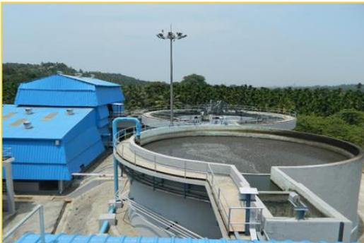
At Gingee, we have established a Water Treatment System in distillery plant, to treat the highly acidic condensate produced during processing of concentrated spent wash. This is treated through Anaerobic Digester and Extended Aeration Tank followed by Clarifier and is used for molasses dilution in Fermentation process.
